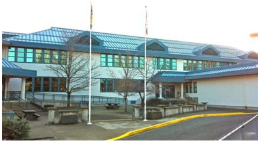
Lake Cowichan Secondary School
